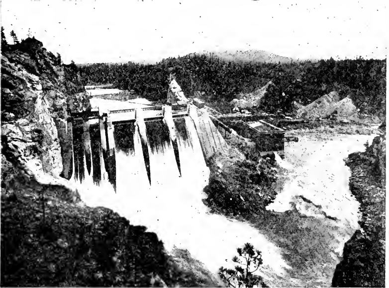
FIG. 50.—Dam of Washington Water Power Company, Showing Arrangement of Rolling Gates.
